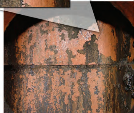
This crack may be small, but it could open as wide as 1/4 inch when the flue is overheated.
