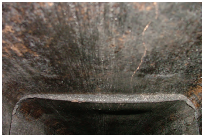
A crack like this can allow deadly gases to leak into the home, and can open the way for a chimney fire to turn into a house fire
