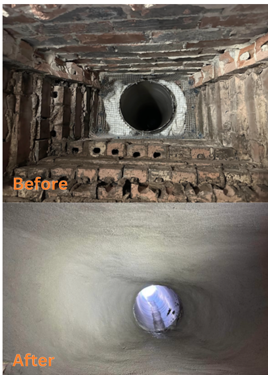
Smoke Chamber Repair
