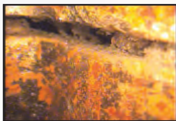
Actual photo of deteriorated mortar joint between flue tiles
