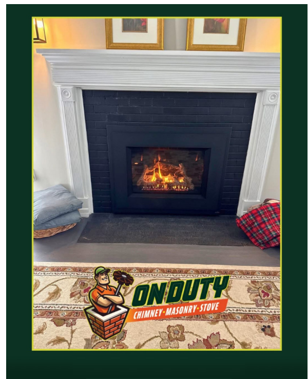
Gas Fireplace Install
