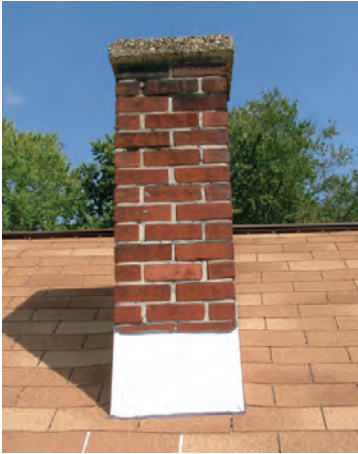
Disintegrating chimney
