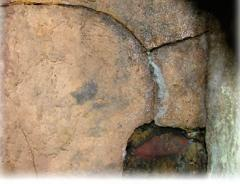
Damaged flue: Notice the moisture and the missing piece of flue tile.
